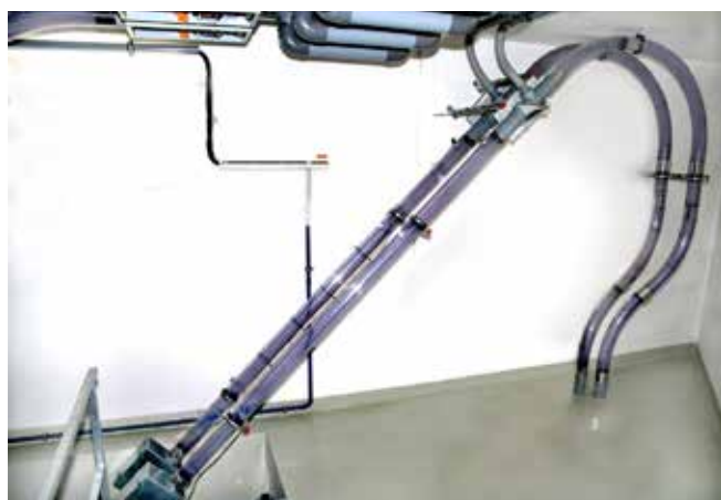
Empty-carrier storage for automatic return of carriers to the home address.
