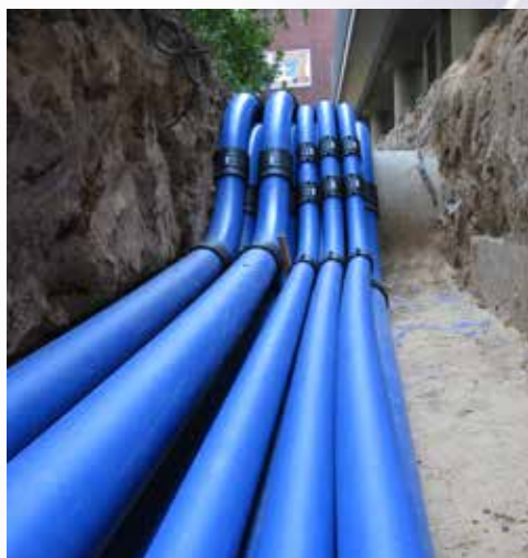
Buildings within a building can also be connected using special PEHD underground tubes.
