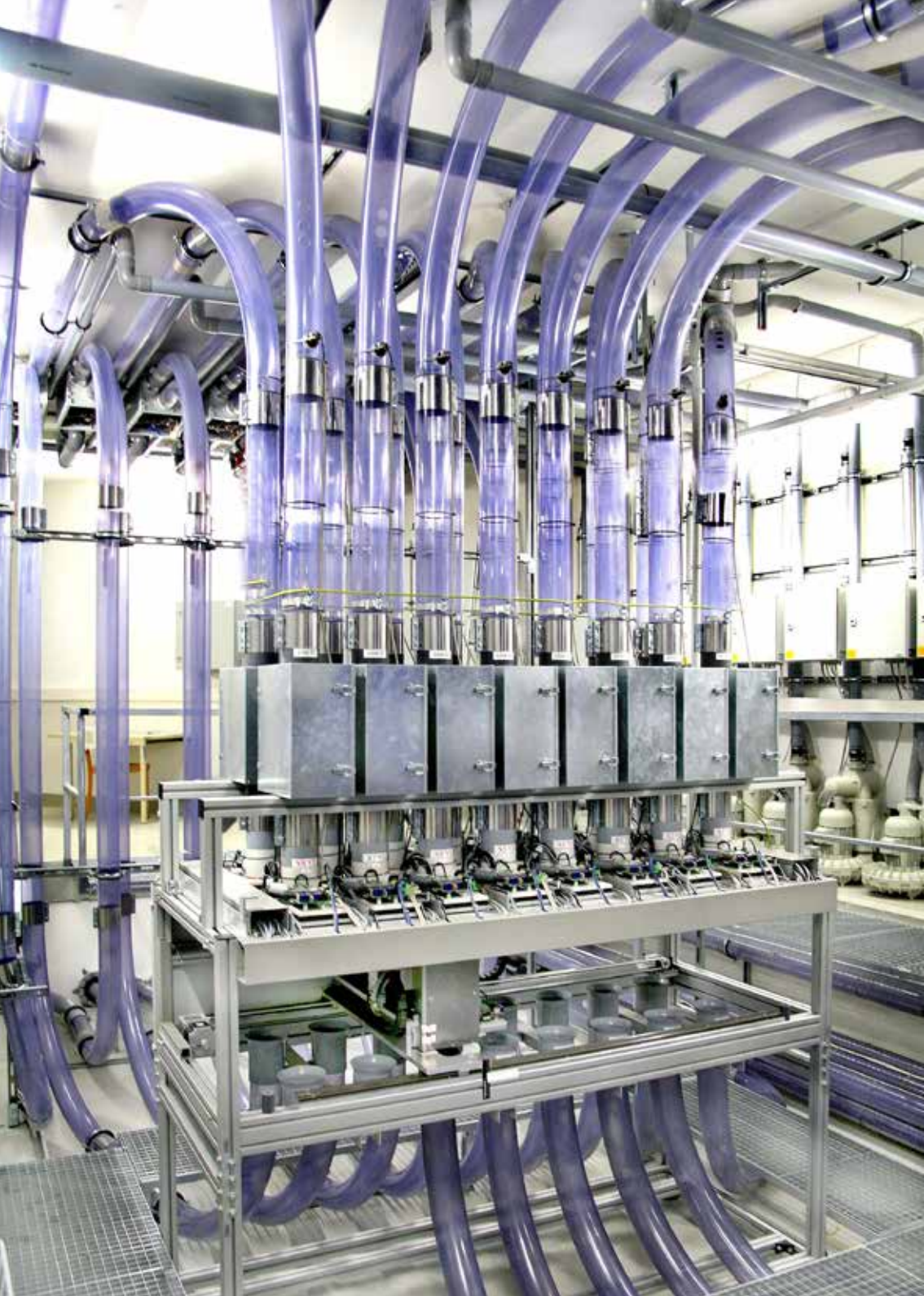
Carriers can be stored above the linear coupler. Carriers can be passed on upward or downward depending on the system.
